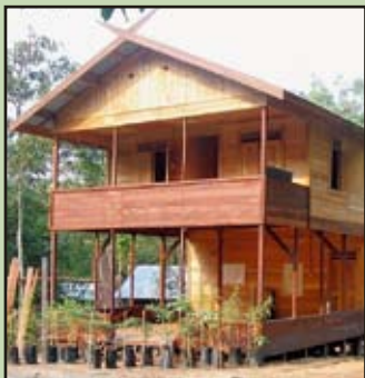
Training centre/guard post in Belantikan
